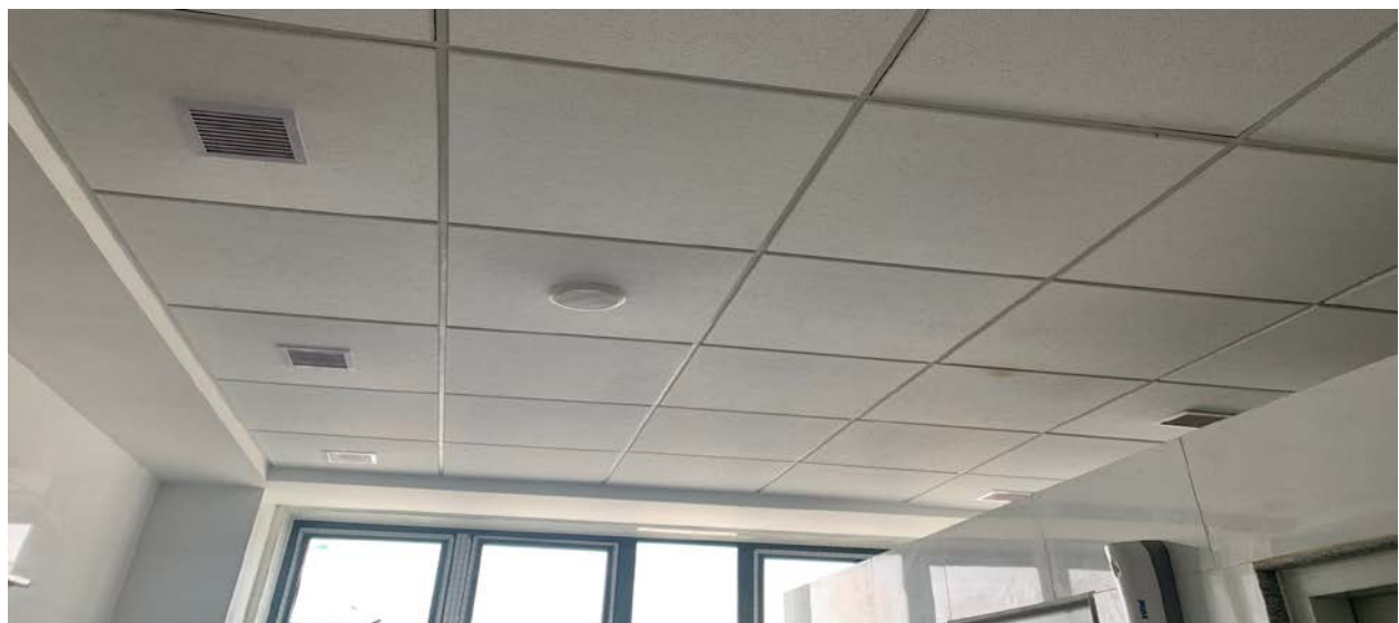
Air circulation duct opening for admin building
