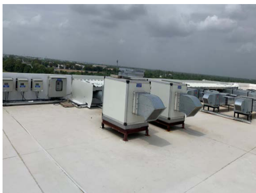
Exhaust outdoor unit for factory
