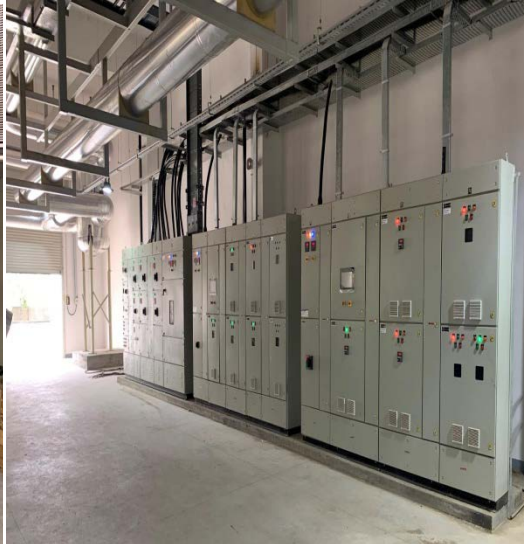
HVAC Electrical Panel
