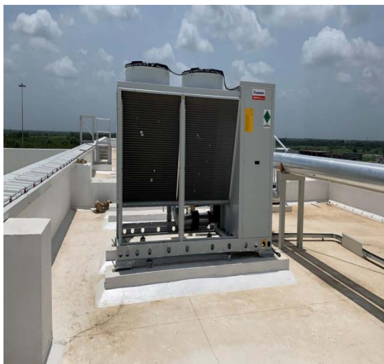
Moulding process water chiller
