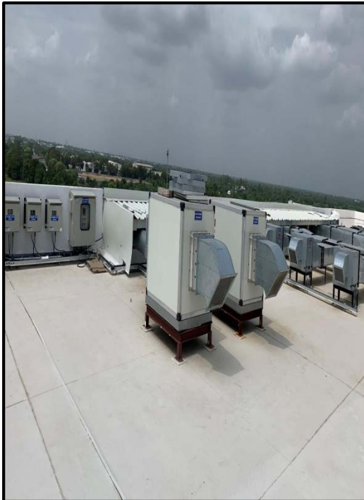
Plant building exhaust fans-outdoor units
