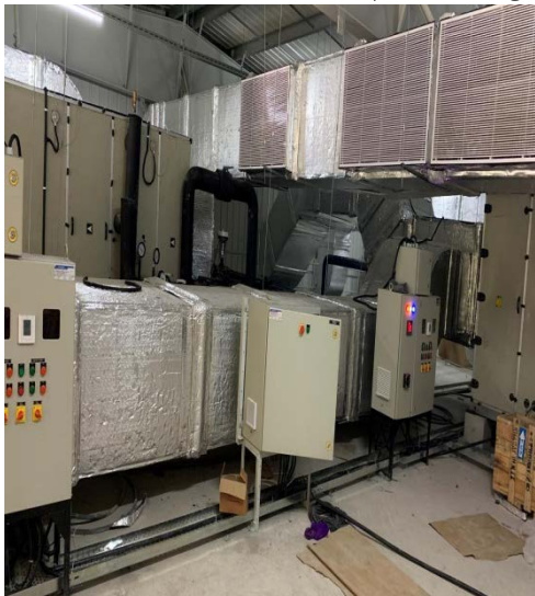
AHU + Panels + BMS Panel
